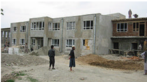
Work proceeds on hospital in early April 2002
